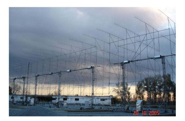
The array not only turns and elevates, but the whole system can be raised and lowered, presumably to help with maintenance. Visit Sam's web site (<a href="www.73.ru">www.73.ru</a>) where you'll find a short video showing the array performing all its moves.
